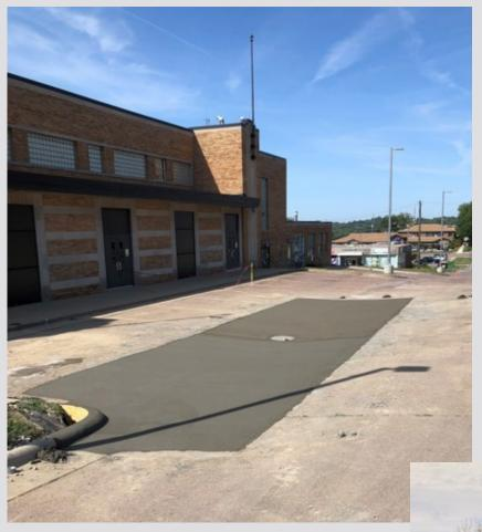
A local apartment complex had settling issues in the parking lot. MJ Minor diagnosed and dug the area up to find a broken storm drain.
